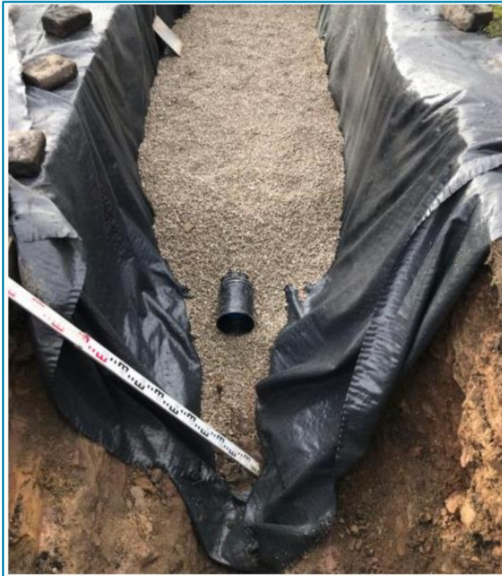
Figure 6-13: Typical Rain Garden Construction
